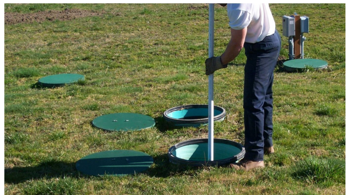
Septic Inspection in Progress
